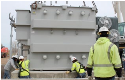
Workers set the transformer on the pad.
