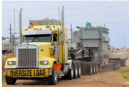
The 110,000-pound transformer is delivered to the substation.
