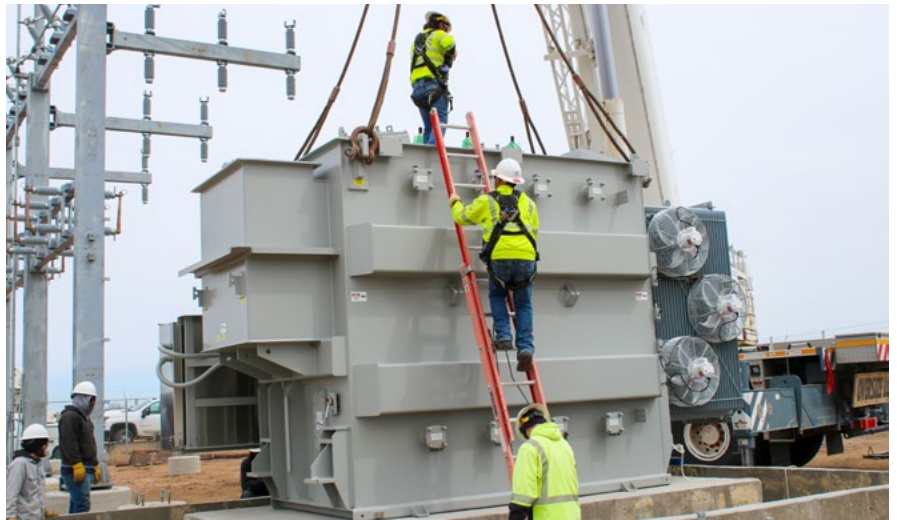
Workers unhook the crane rigging after the transformer is in place.
