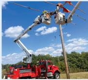
Victory linemen learned the proper procedures for positioning, covering up, changing layouts and switching out structures when working with live lines.
