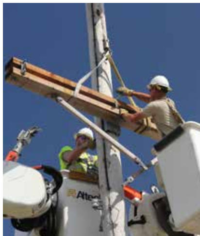
Kade Henry (left) and Jeremy Elling place a new crossarm on a pole.
