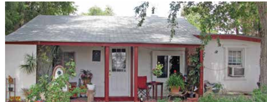
As a result of a WAP inspection, the Garcia family replaced a water heater, which saved them money and saved their lives.
