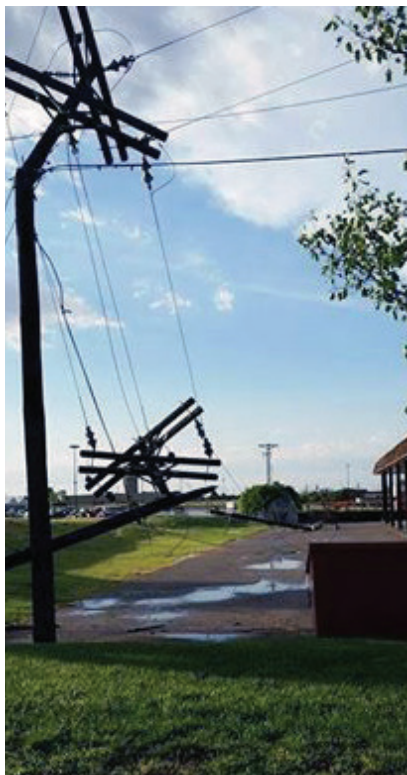
Wind blew down lines and poles in residential and commercial areas of Dodge City.
