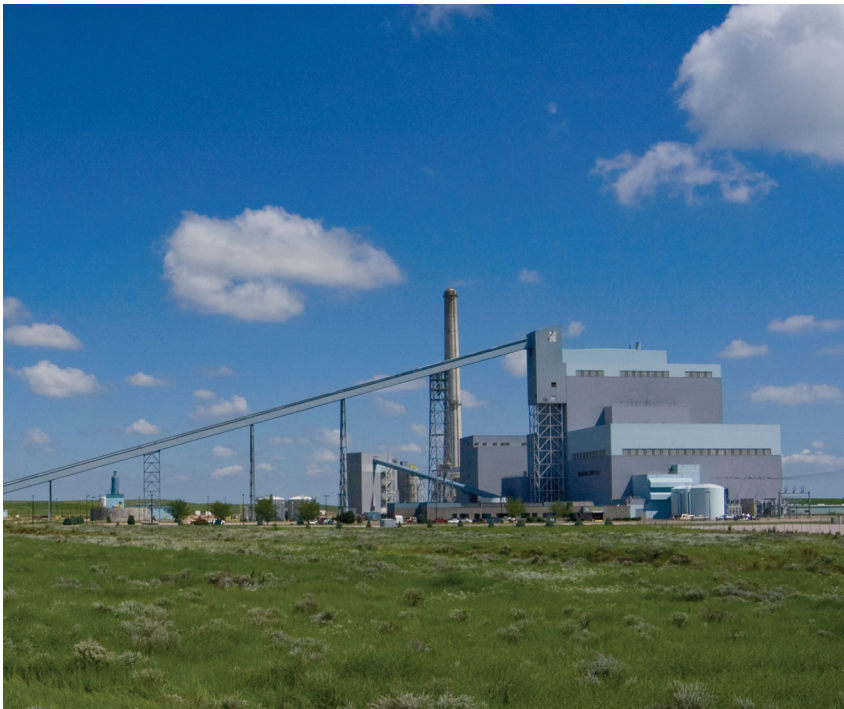
Holcomb Station for Sunflower Electric Power Corporation supplies Victory as one of the G&T plants.
