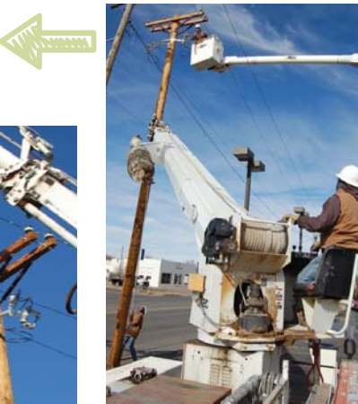
After the hole was dug, Woods lifted the pole into place while Stormont navigated the new pole around the existing wires and Ledford steadied the pole from below.
