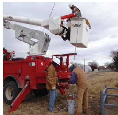
Crews prepared and hung a temporary transformer so power could be rerouted. This allowed the crew to safely replace the poles and equipment without the surrounding homes and businesses losing power.
