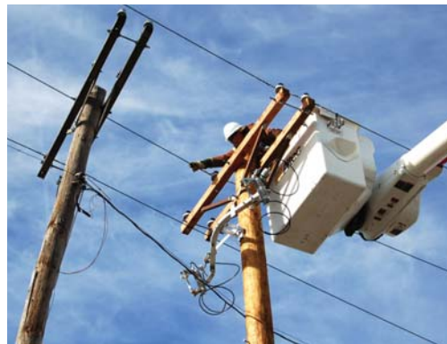
Crews prepared and hung a temporary transformer so power could be rerouted. This allowed the crew to safely replace the poles and equipment without the surrounding homes and businesses losing power.
