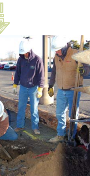
Replacing poles is not always an easy task. In this instance, there was a 12 inch gas main less than a foot away, so the linemen dug the top of the hole by hand and located the gas main before using the auger.
