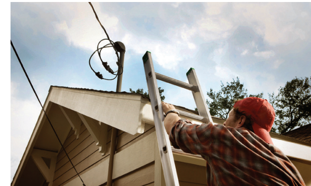
Ladders placed too close to power lines become dangerous conduits of electricity.
